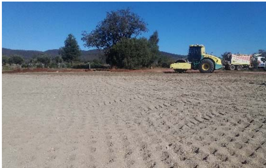
Earthworks at The Living Classroom
