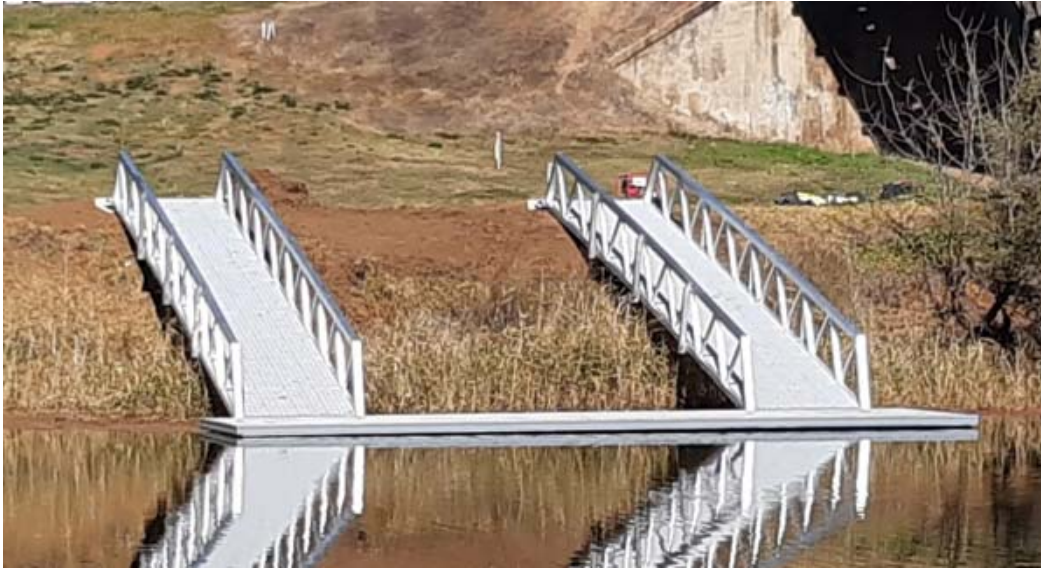
Pontoon upstream of Gwydir River Bridge
