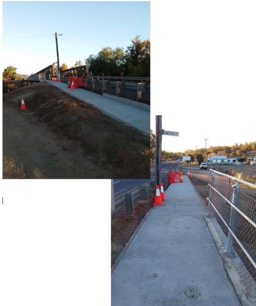
Campbell Bridge, Bingara
