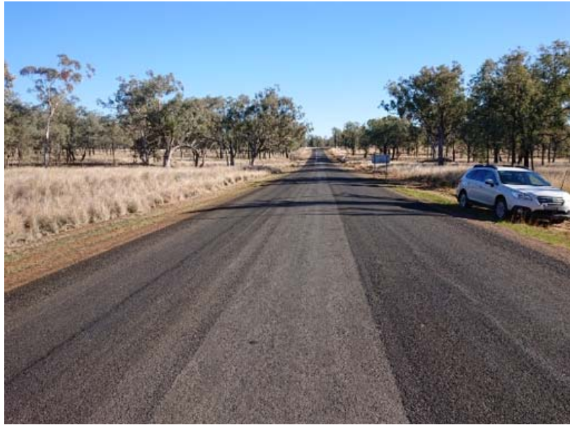
Newly widened formation of on North Star Road
