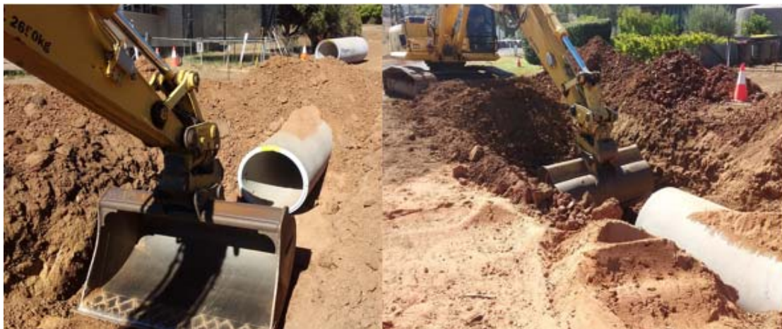
New stormwater main running from Maitland St to Spring St, Bingara
