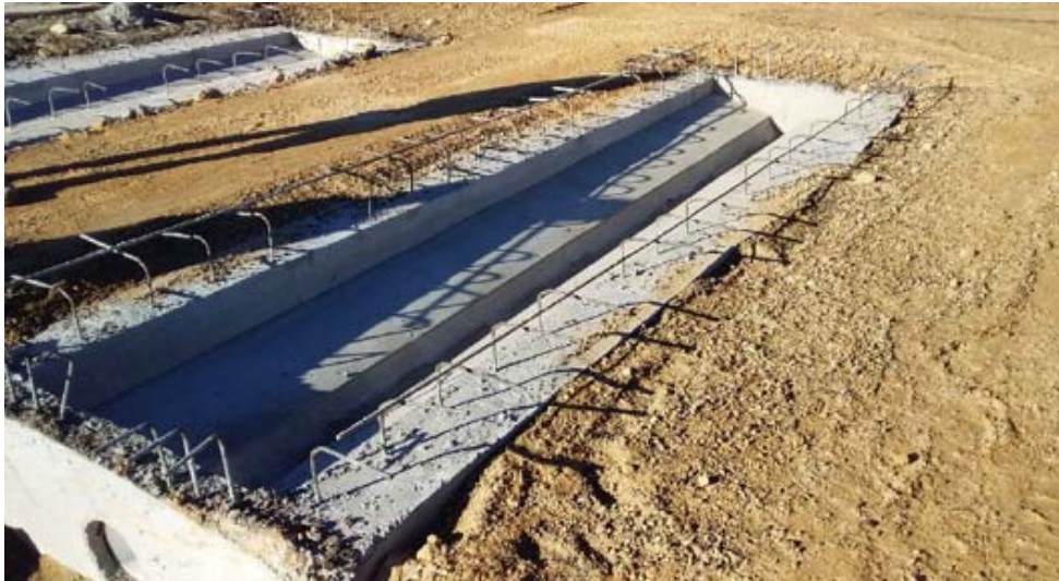
Base of Effluent Dump Points – Warialda Truck Wash
