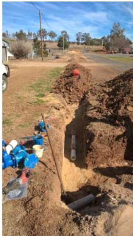
South Street water main extension
