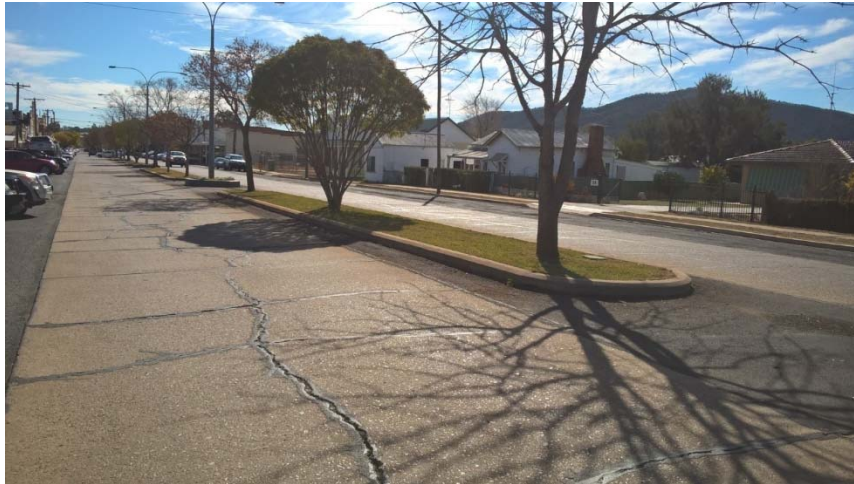
Centre garden turf in Maitland Street, Bingara
