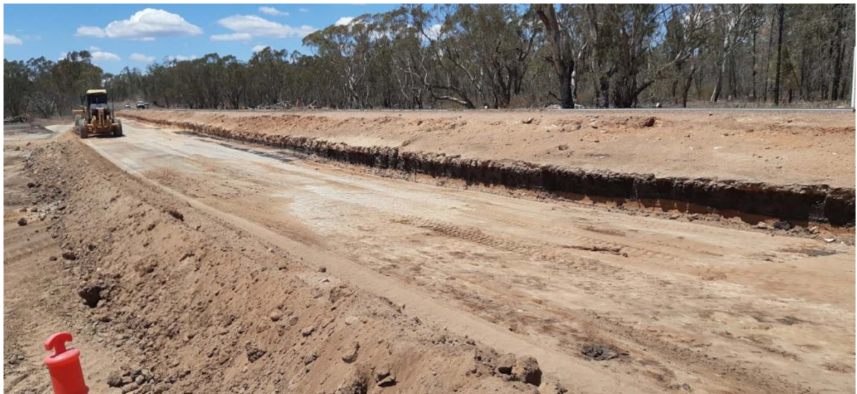
Construction crews have cleared the footprint and started to lay material for the intersection.
