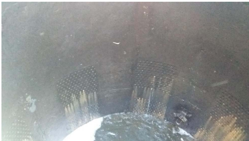
Bingara river intake chamber with restricted flow
