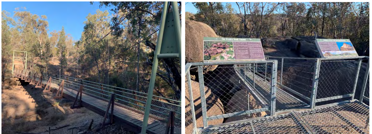
The footbridge and viewing platform at Cranky Rock
