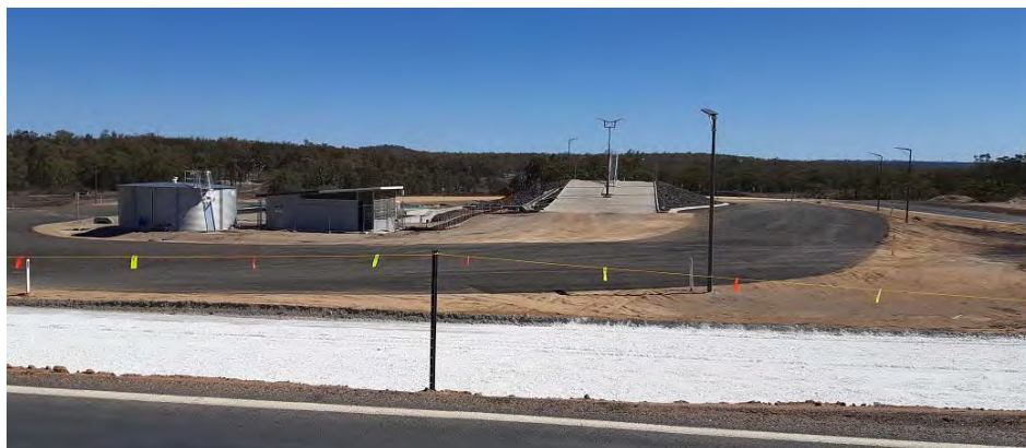
Truck Wash Site, Warialda
