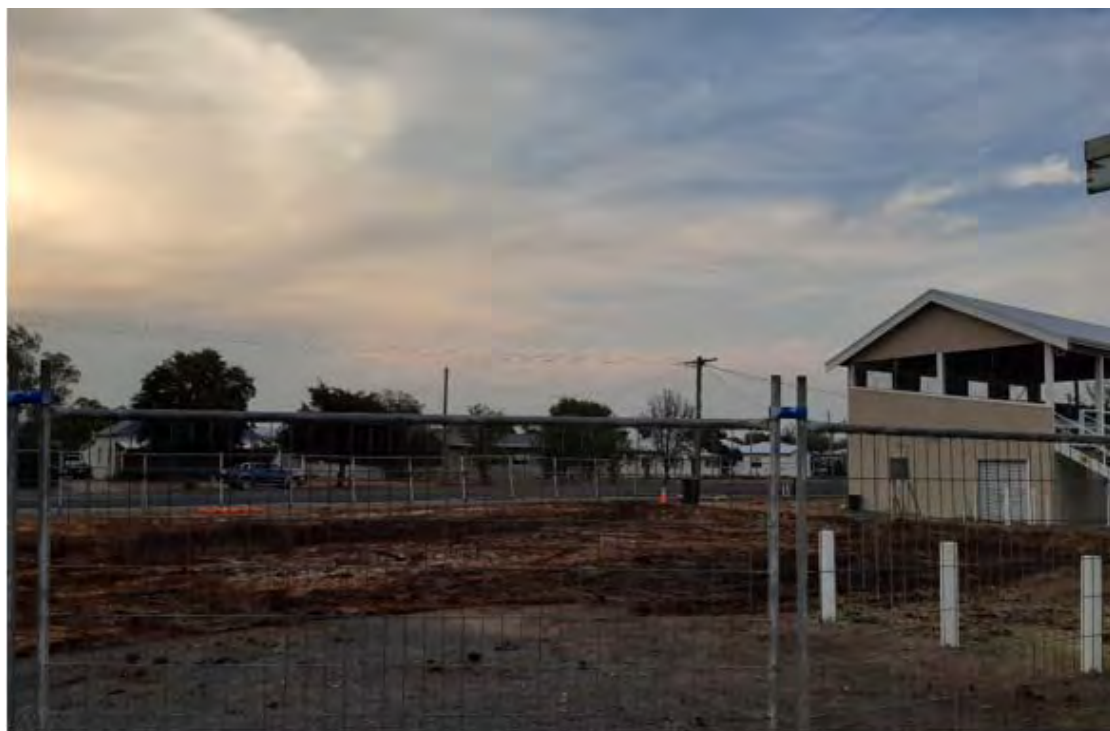
Removal of old amenities at Gwydir Oval
