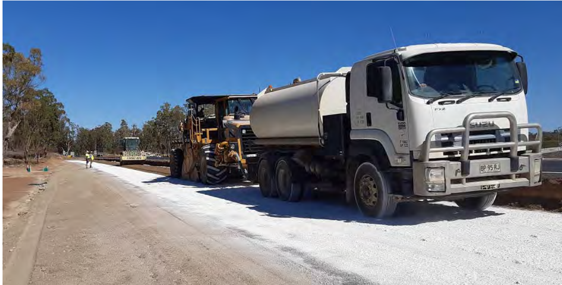
Stabilising at the HW12 Intersection, Warialda
