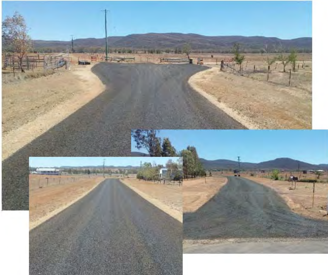
Completion of Park Lane, Bingara
