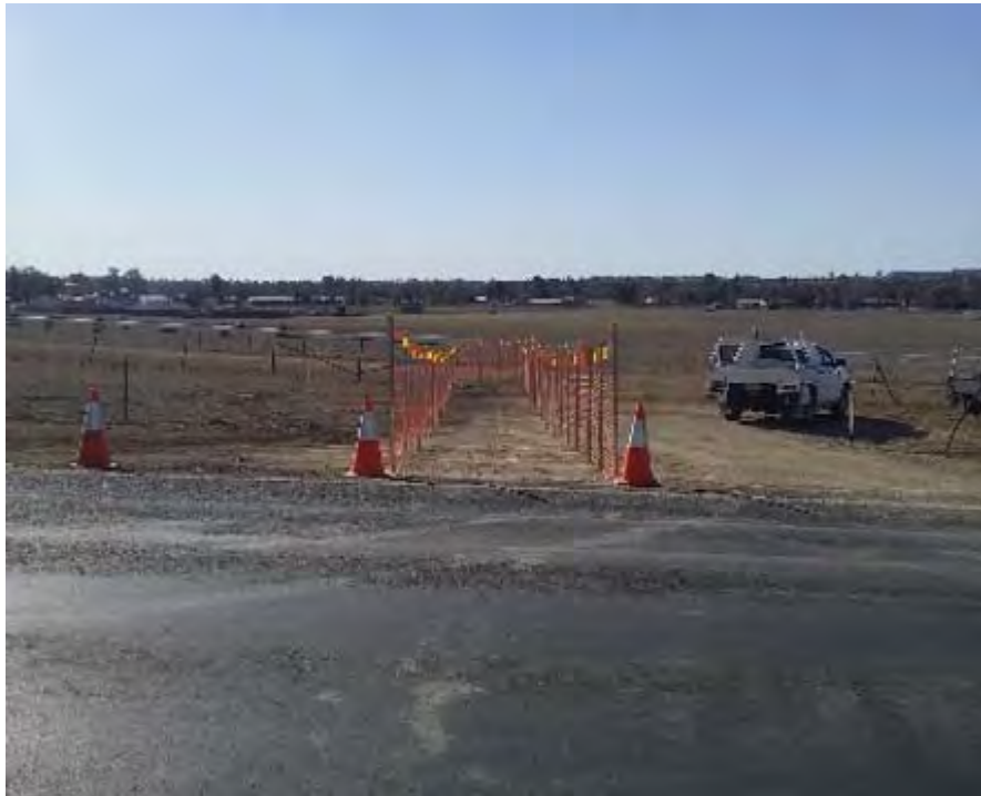
Water Staff built an access for cars and a safe pedestrian walkway for the Pulse Festival Plant and Workshop
