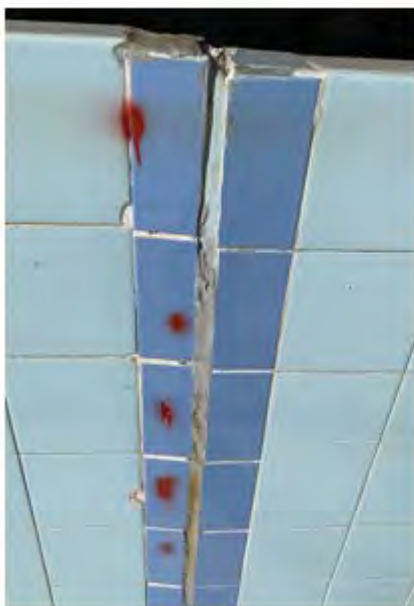
Damaged tiles at Bingara Swimming Pool
