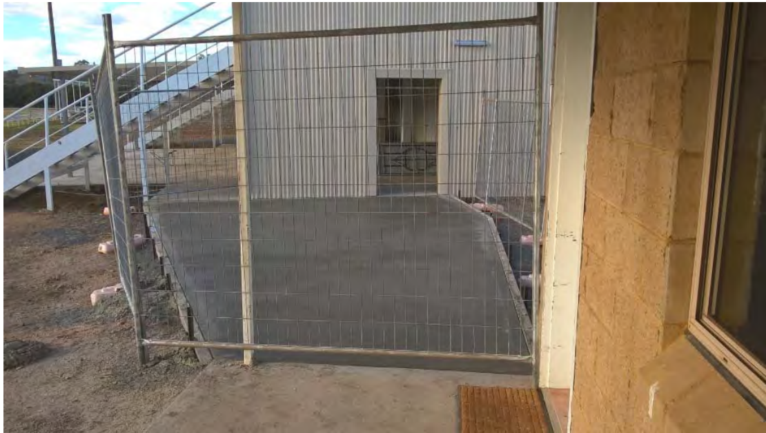
Footpath near Gwydir Oval canteen
