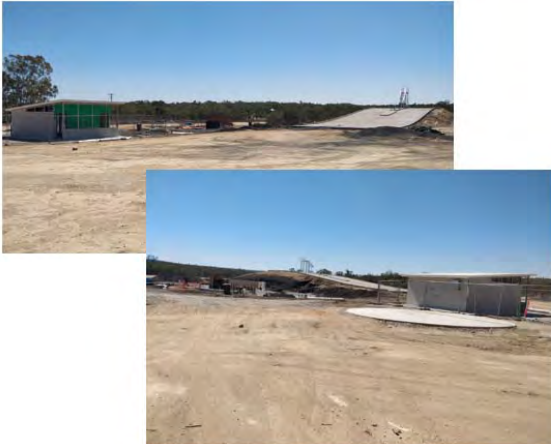
Warialda Truck Wash, amenities block and tank pad
