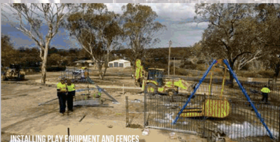
INSTALLING PLAY EQUIPMENT AND FENCES
