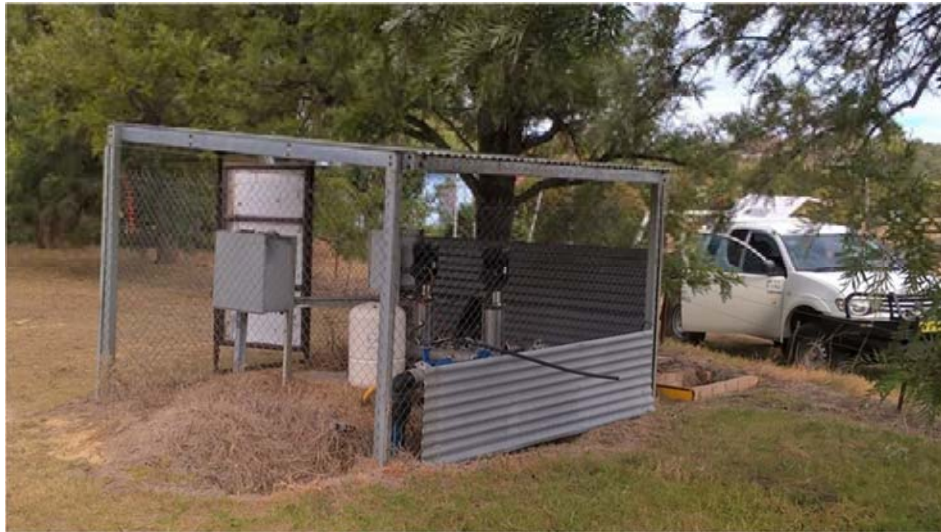
Golf course variable speed effluent pumps
