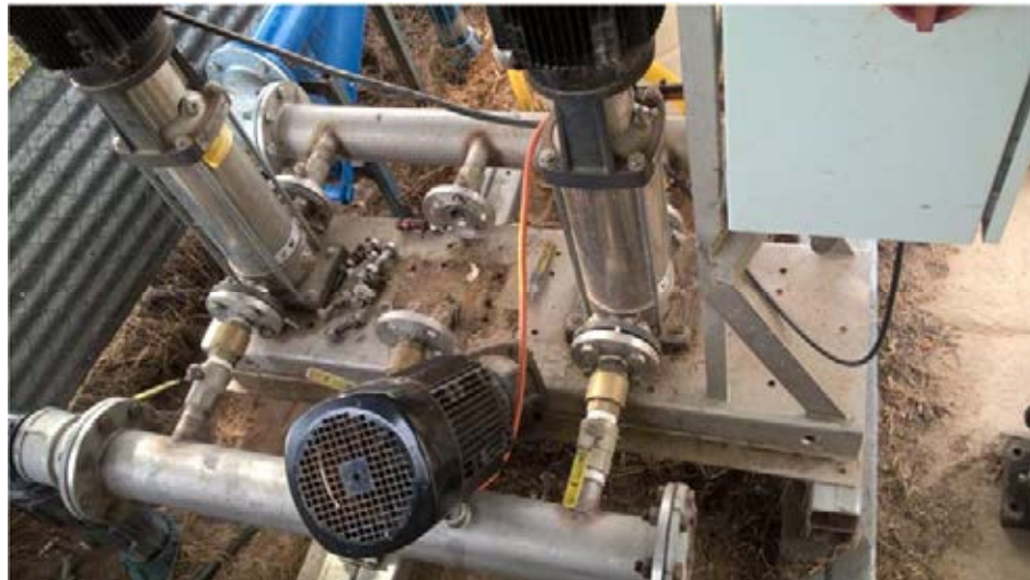
Pump 2 – out of service
