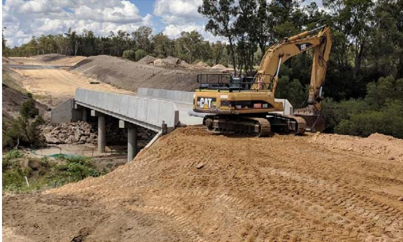
Two pavement layers have been laid between the Gwydir Highway and Reedy Creek with the third and final layer in the process of being carted.
