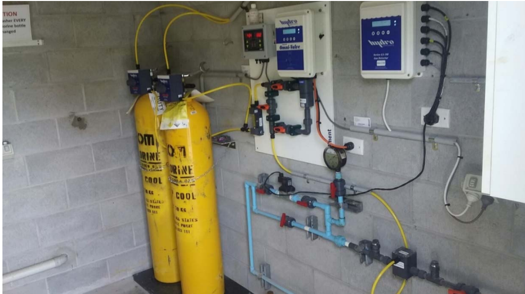
Bingara chlorine gas disinfection
