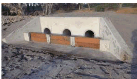
Figure 4: Typical Control Weir from a Sediment Basin
