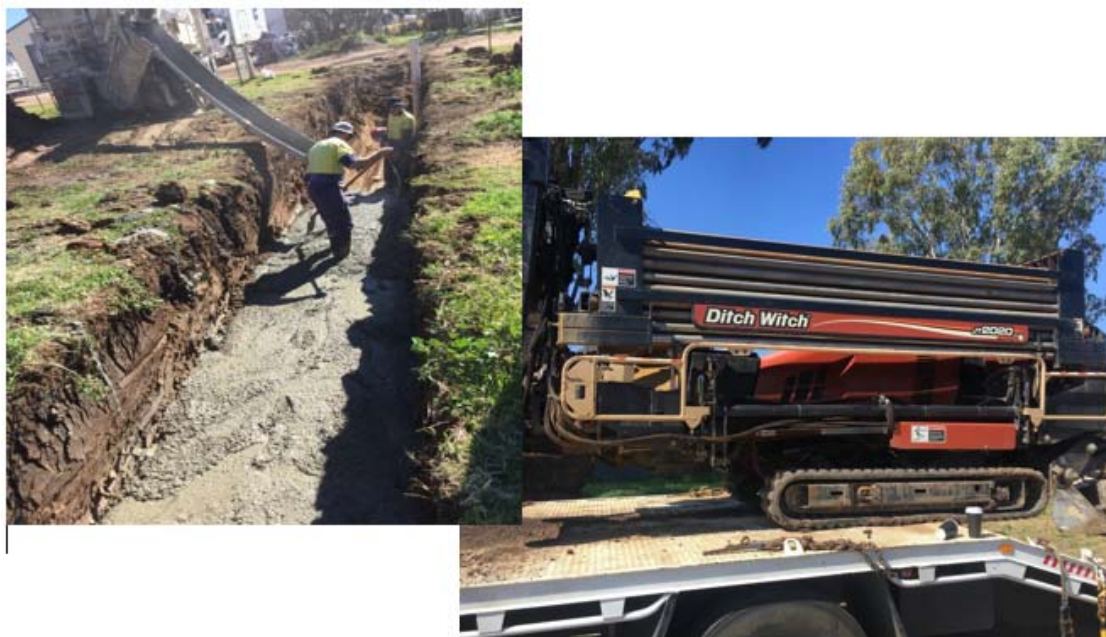
Sewer Main Encasement and Horizontal Boring Unit
