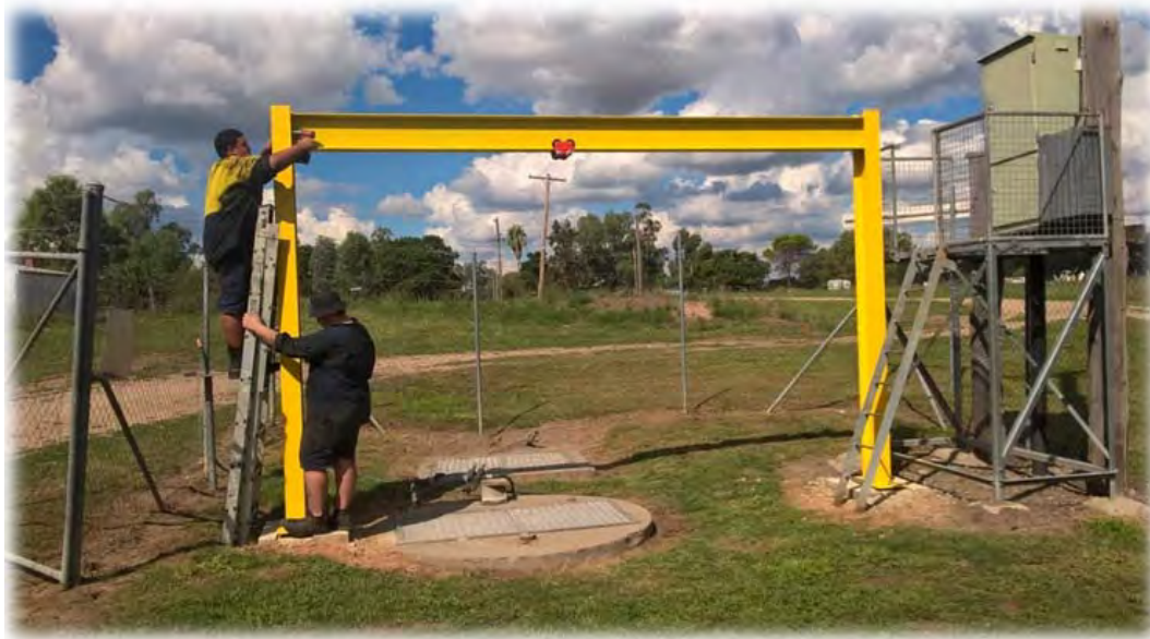
Installation of sewer pump station gantry
