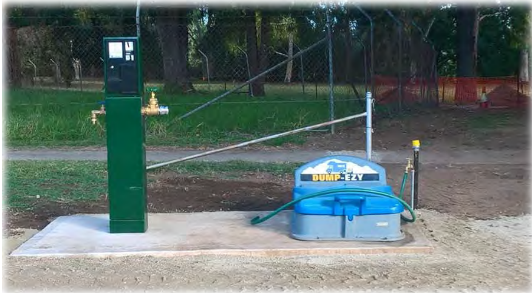
Coin operated Standpipe and dump point
