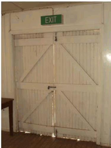
Emergency Exit door padbolted and without panic bars
