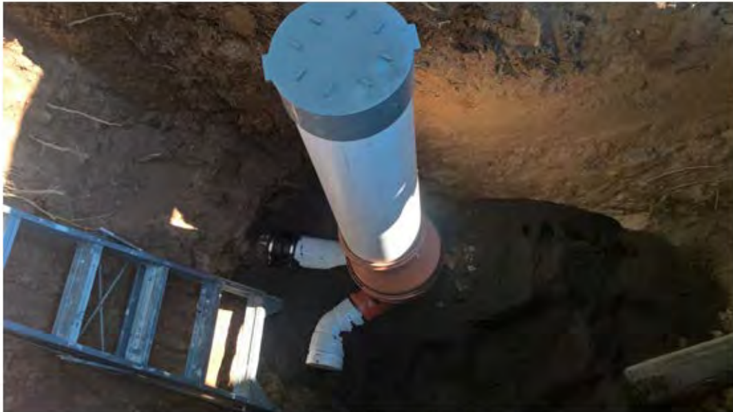
New sewer connection and access pit
