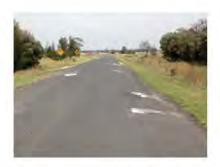
The road meets the minimum carriageway width in the NSW Route Assessment Guide – freight route investigation levels (30 October 2012) for vehicles from 20m to 36.5m for straight unsealed roads with an AADT between 1 and 100 of 7.0m for two-way travel.
