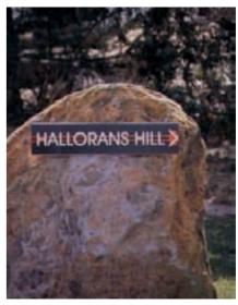
Cut or flat boulders can be installed into the pathway edge and act as vehicular barriers. Signage can also be incorporated into the pedestrian faces.
