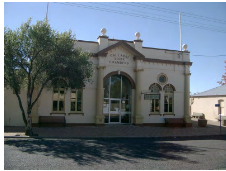
Warialda Council Chambers
